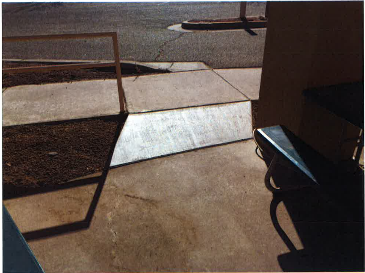
Senior Center: Replace vaulted sidewalk (obstruction) – constructed by City Forces 2017.
