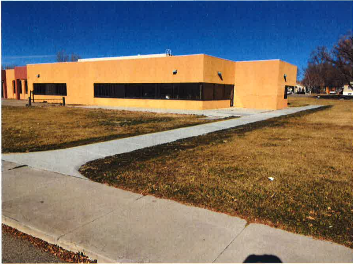
Cultural Center/Fitness Center: AR to East Door of Fitness Center-constructed by City Forces 2017.
