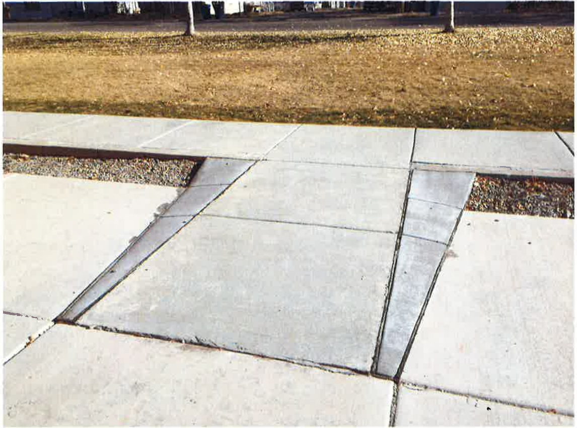
Cultural Center/Fitness Center: AR to East Door of Fitness Center-constructed by City Forces 2017.
