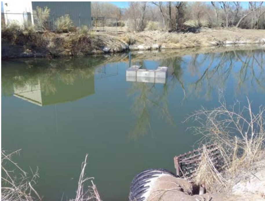
Floating suction device while pumping 1,170 gpm constructed by Public Works.
