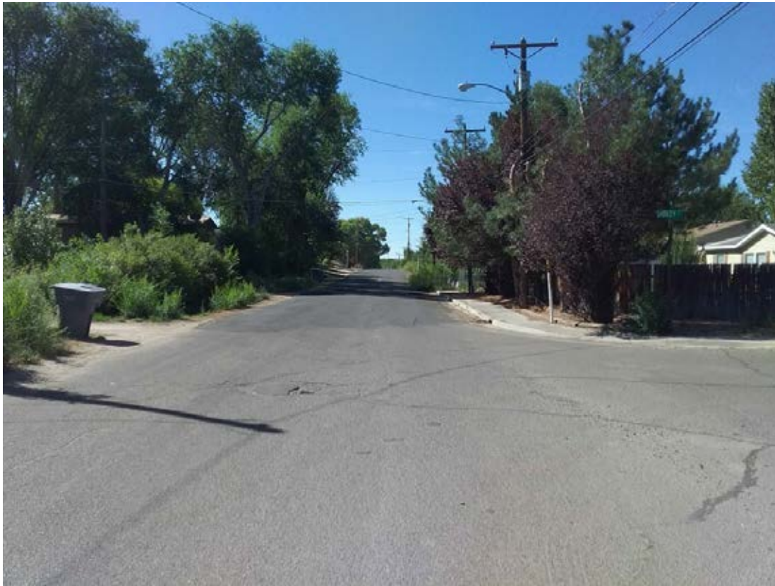
Saiz Lane sewer repair asphalt patch, looking south from Shirley Street.
