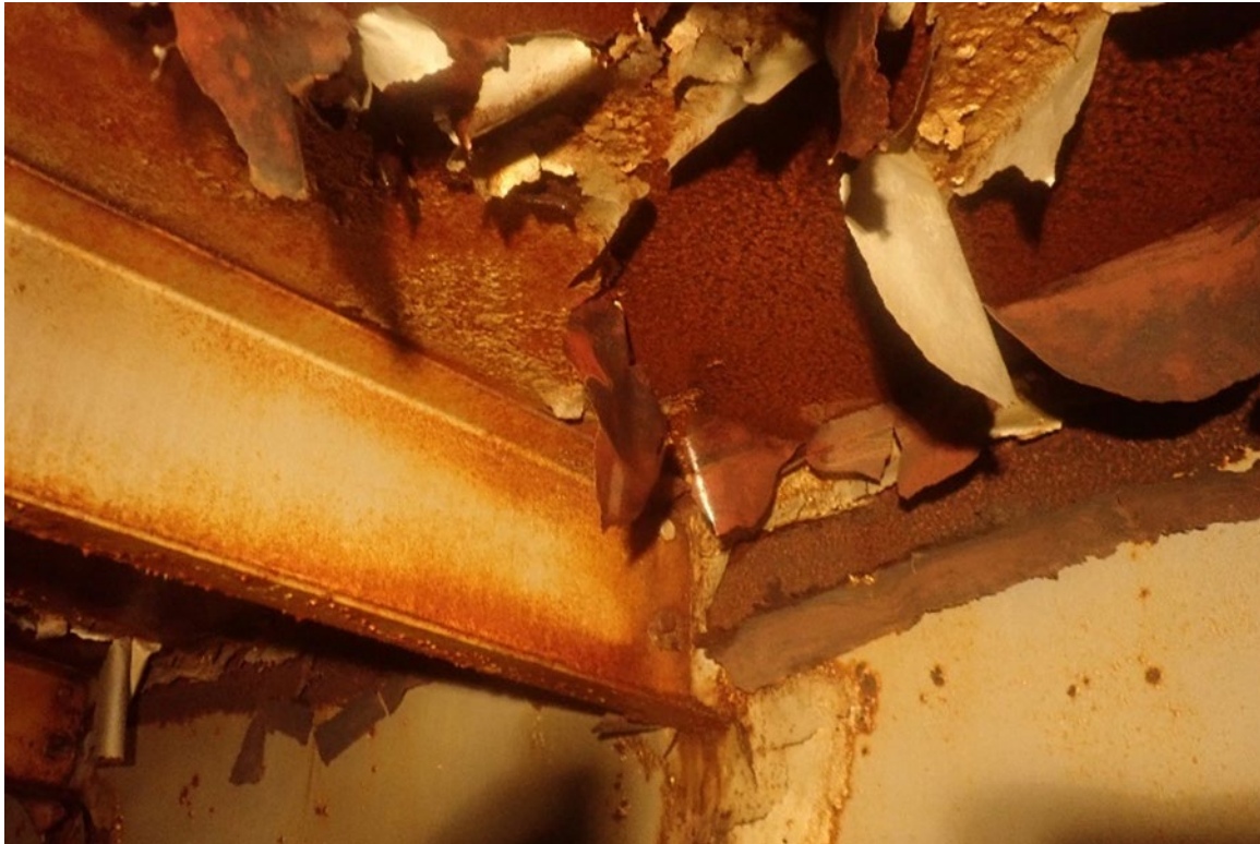
Interior coating where the roof joins the shell.
