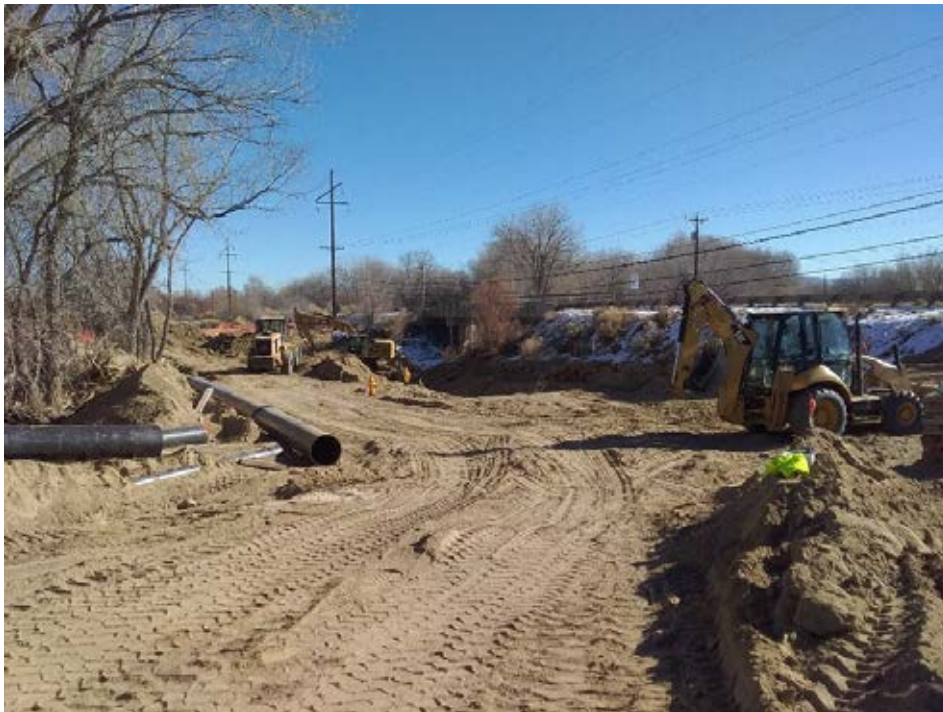
Phase I utility relocation by Halo Services in February 2021.
