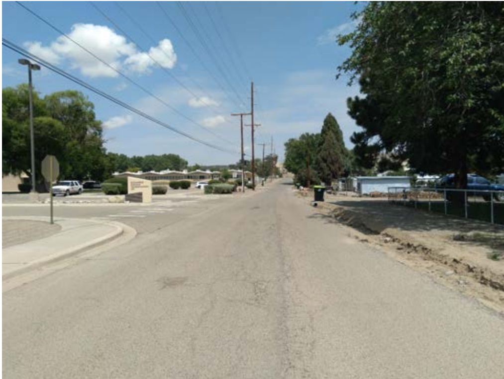
View looking north showing poor drainage features and no continuous sidewalk.
